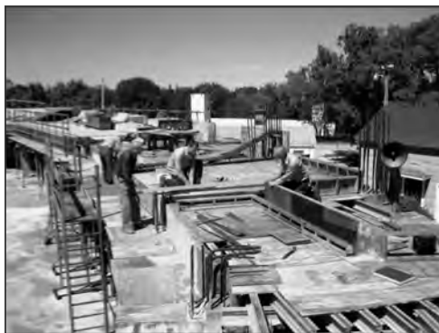
Setting Up Shoring and Forming for the Fifth Pour
